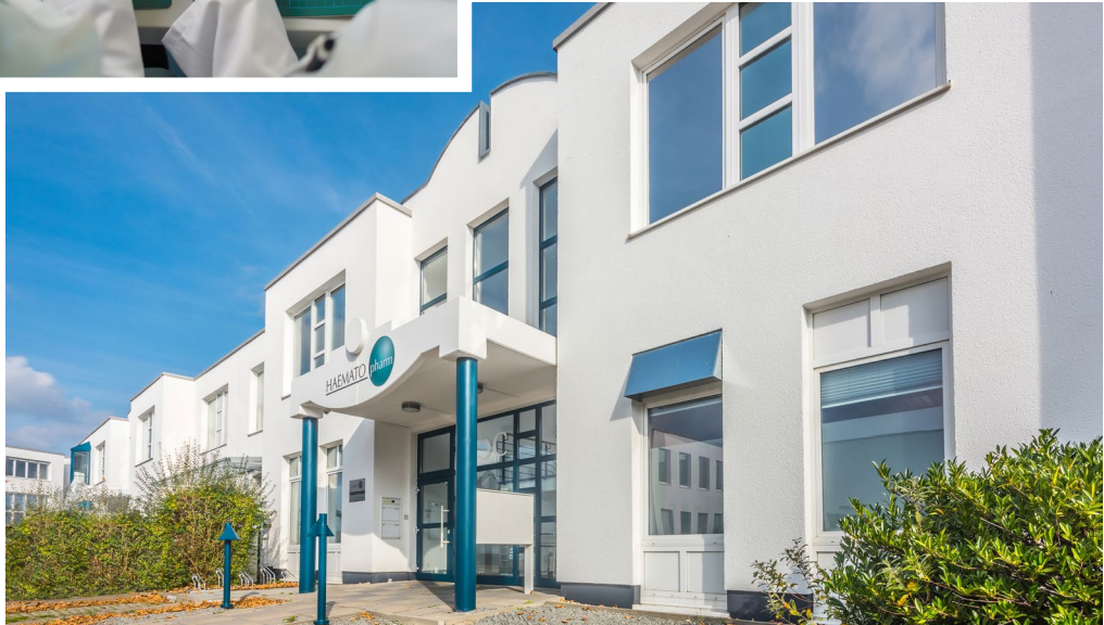
Main building of HEAMATO AG
