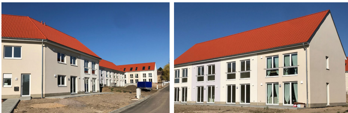
Construction project Schkeuditz (sample photos - non-binding visualizations)
